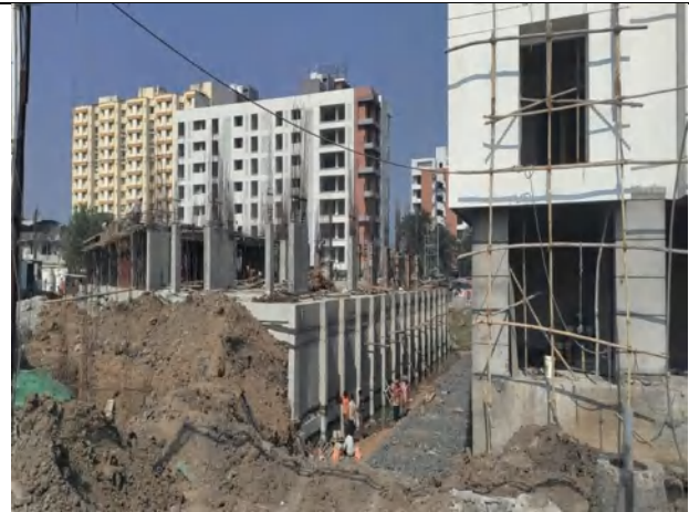
Civil work of commercial building Pramukh Orbit 3 is going on
